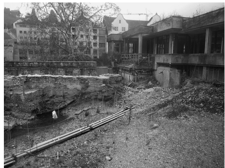
Fig. 2 Thermal Baden under construction
